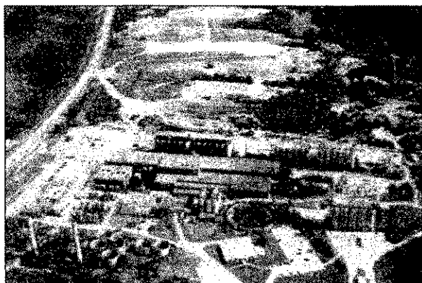
View of Lehigh Cement property looking north
