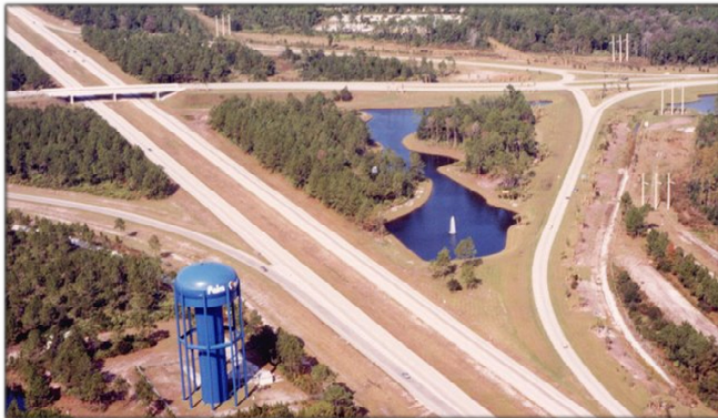
I-95 Interchange at Palm Coast Parkway
